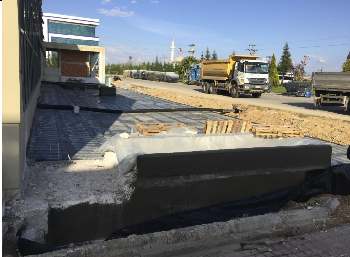
UNDERGROUND RANGE CONSTRUCTION
