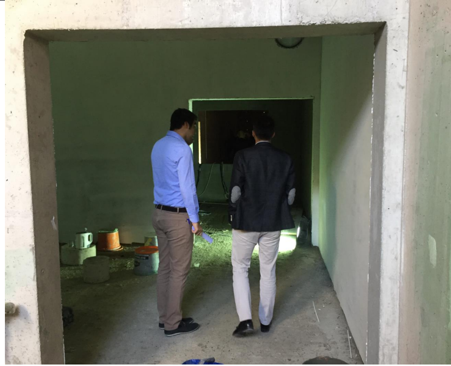
MEETING ROOM. THIS IS THE ENTRANCE TO RANGE
